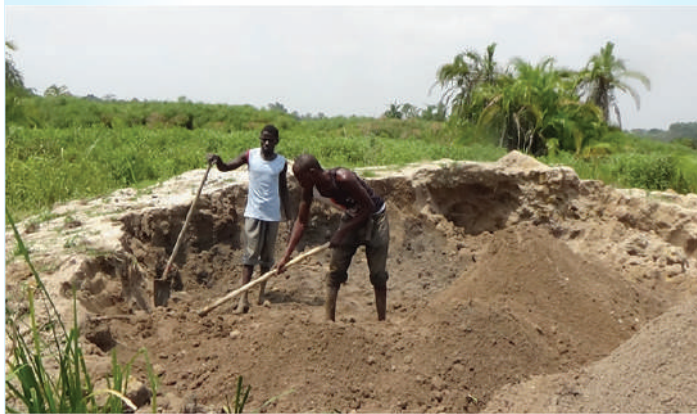
Youths at Lugala excavating sand using hoes and spades
